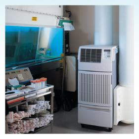
**Cost-effective and flexible:** For areas the main HVAC system does not reach, or when the main system is switched to heating mode.
